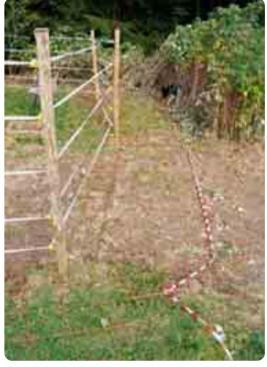
Photo 12 - Electric welded mesh to prevent digging, tried out experimentally at the base of electric fences (E. Bonapace, APT Forestry and Wildlife Dept. Archives)
